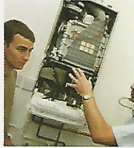
Worcester helps install
