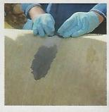
pipes. It can repair long splits and cracks in cast iron, copper, plastic, clay and all other pipe materials, from 15 to 300mm diameter. The product is WRAS approved and can be used to stop pressurised leaks when flow cannot be isolated. **Circle readerlink 252**
