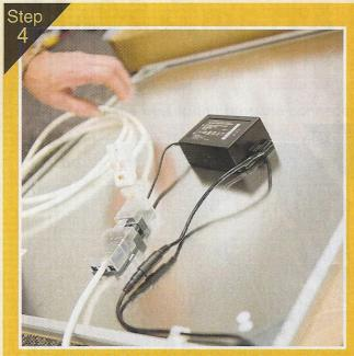
The installation of the driver is simple on the flat panel, thanks to its plug and play function. One thing to remember though is to put the driver in the middle of the fitting when installing it into the suspended ceiling, so that it sits away from the LEDs (which emit some heat when in operation).
