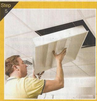
When installing the Kurve panel into the suspended ceiling however, it is simply a matter of connecting it to the inline socket, no care needs to be taken with the driver as this is integral to fitting already.
