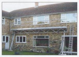
safety handrails and end rails are then attached. The system is tested to full European safety regs.
